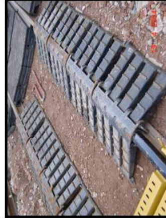
Ramp section engaged on to the rail.
